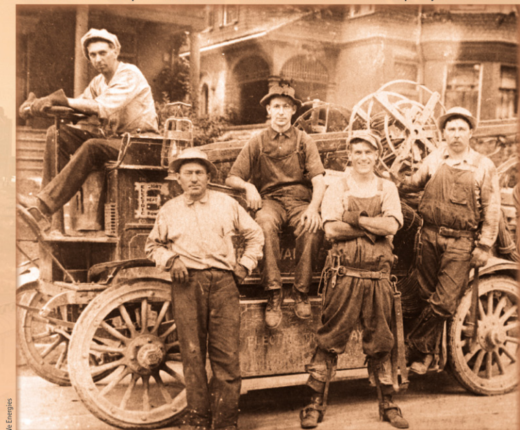
Overhead line repair crew for the Wisconsin Electric Company, 1930s.
